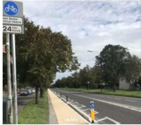
**Figure 5 - Extruded concrete kerb , Griffith
