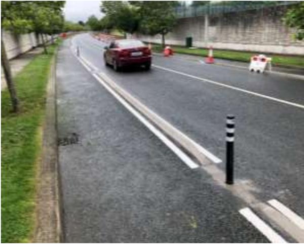
**Figure 4 - Extruded concrete kerb
