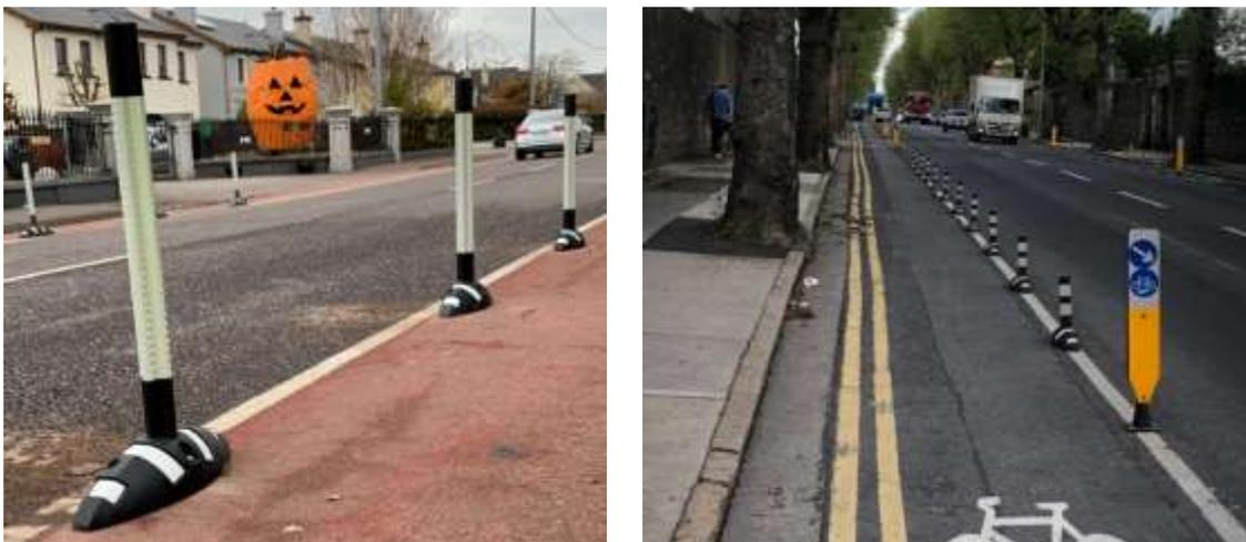
**Figure 7 - Tiger Wand Cycle Lane Separators**
